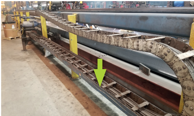
Installation in a cable carrier system used with a longitudinal seam welder
